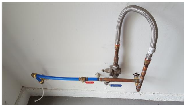
5.2 Item 2(Picture) Informational photo of water shut off at garage.
