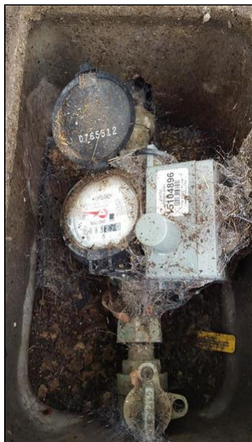
5.2 Item 1(Picture) Informational photo of water meter and shut off at curb.
